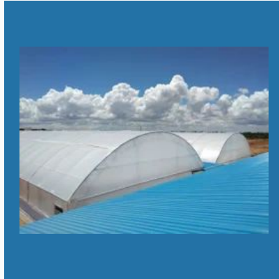
Poly House Doom Structure
