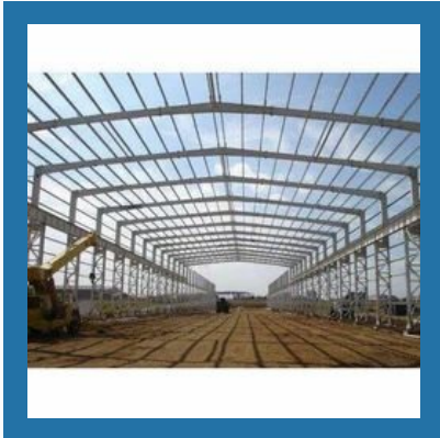
Structural Roofing Service
