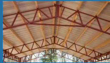
Steel Roof Trusses
