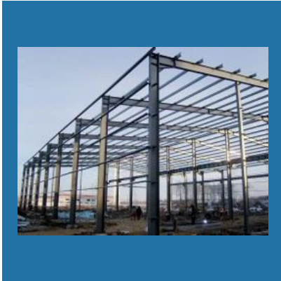
Steel Structure Building
