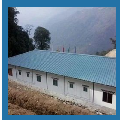
Construction Site Office
