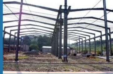
PEB Industrial Roofing Services
