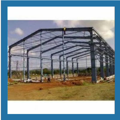
Steel Framed Buildings
