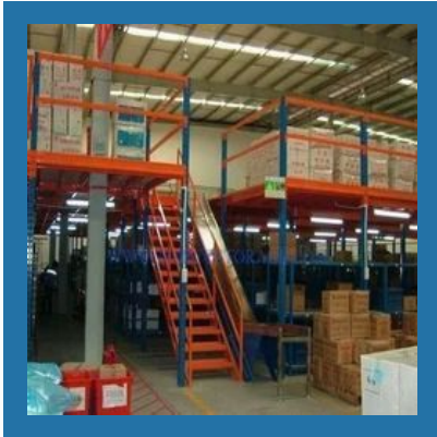
Prefabricated Mezzanine Floor
