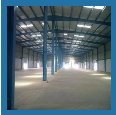
Warehouses Steel Structure
