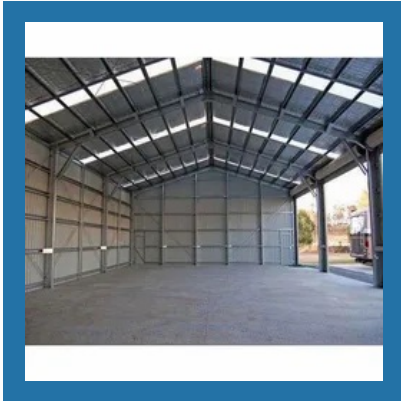
Prefabricated Factory Shed
